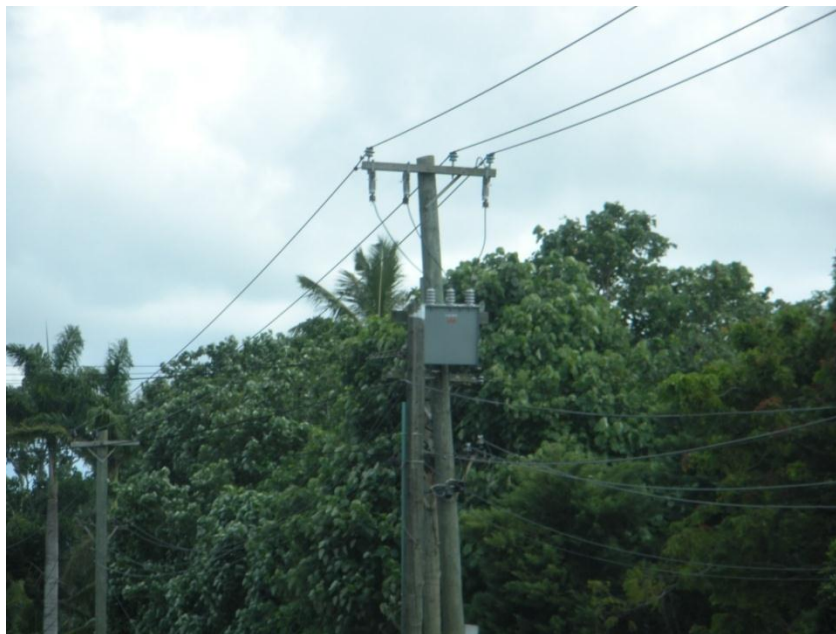
Figure 9 - Typical Distribution Pole with Transformer
