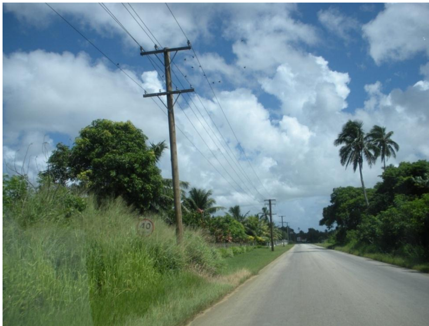
Figure 8 - Typical TPL 11 kV Distribution Line
