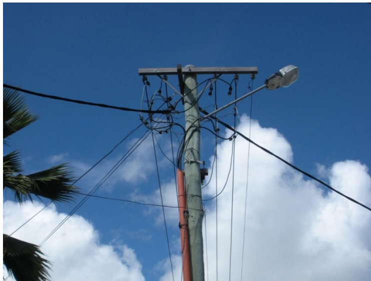
Figure 11 - Distribution Pole Showing Low Voltage Wires
