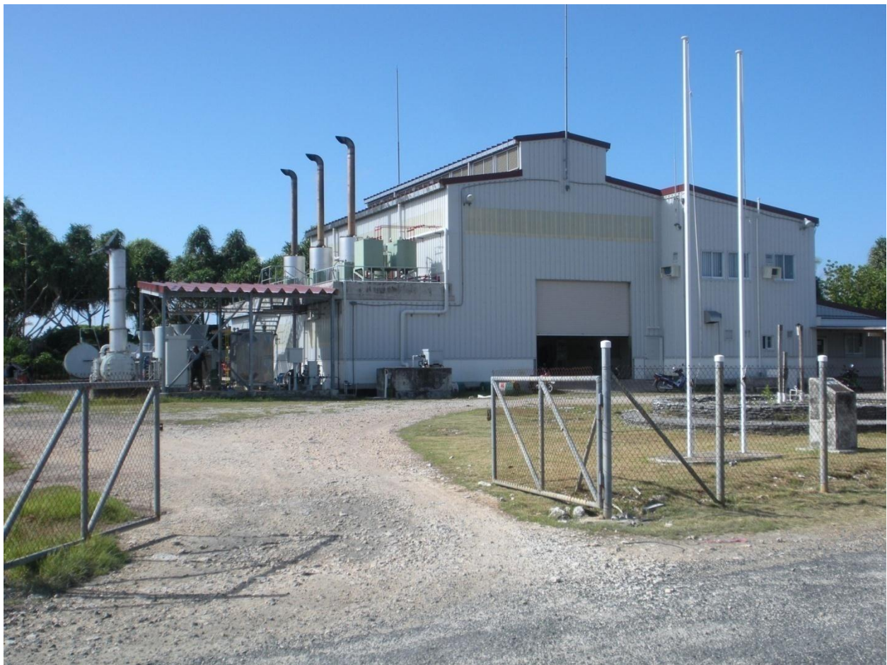
Figure 1 - Power Station Building (as Viewed from Gate)
