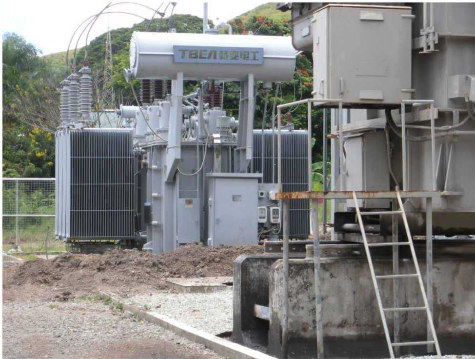
Figure 6 - Sample POM 66 / 11 kV Substation
