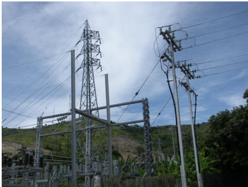
Figure 7 - Sample 66 kV and 11 kV Dead-end Structures at POM Area Substation
