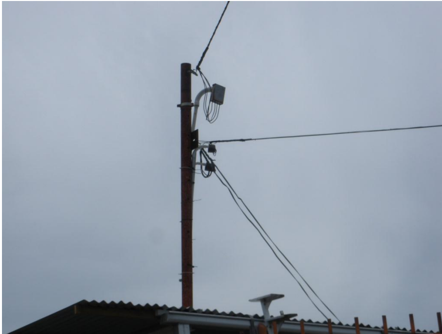
Figure 9 - Sample POM Area Service Wire Assembly
