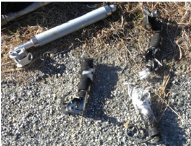
Fig. 8: A common full-range drop-out fuse with a polyurethane fibreglass enclosure. It burnt out under the fault and caused a local bushfire. The only remaining part was fibreglass (Note: photo courtesy of an NZ distribution company)
