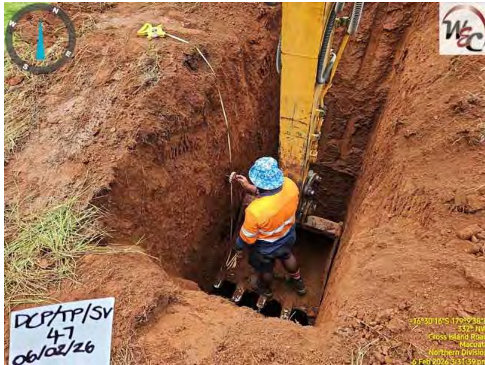
Photograph 14: Shear Vane tests being carried out by the Engineering Technician at Test Location TP 47.
