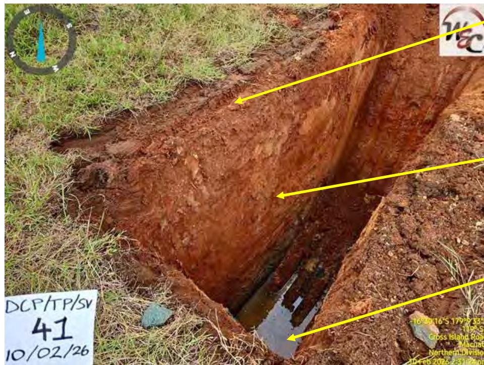
Photograph 9: Photograph indicating generally dark brown Silty CLAY, topsoil (shallow depth), Silty CLAY material which was extracted with an excavator (TP 41) which contained some quartz and minor rootlets with water table encountered.
