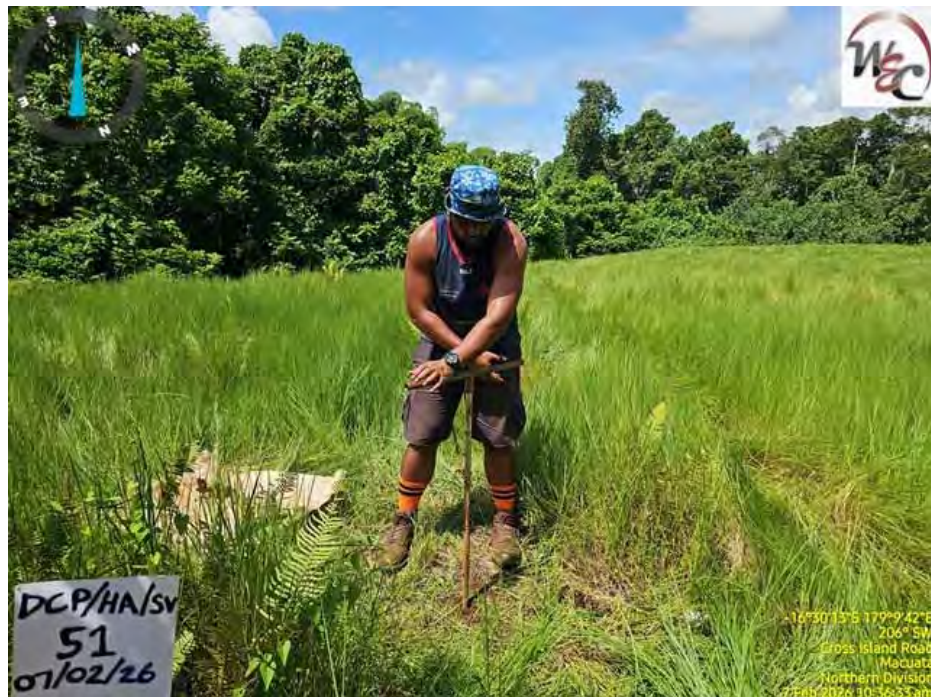
Photograph 13: Hand Auger tests being carried out by the Engineering Technician at Test Location HA 51.
