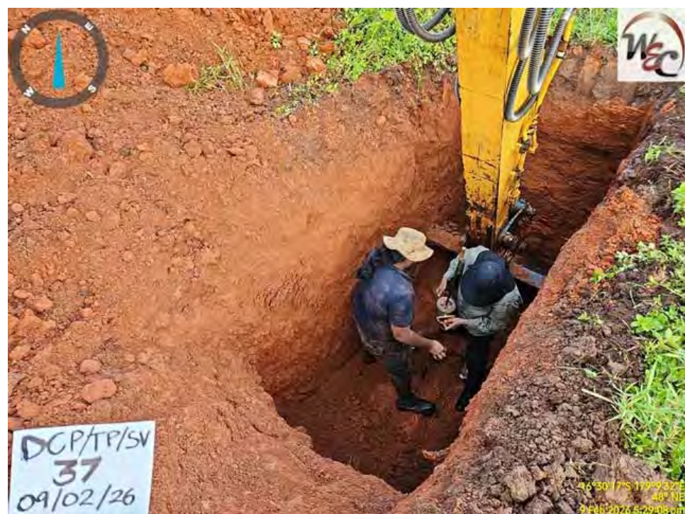
Photograph 15: Dynamic Cone Penetration test being carried out by the Engineering Technician and Graduate Engineer at Test Location TP 37.
