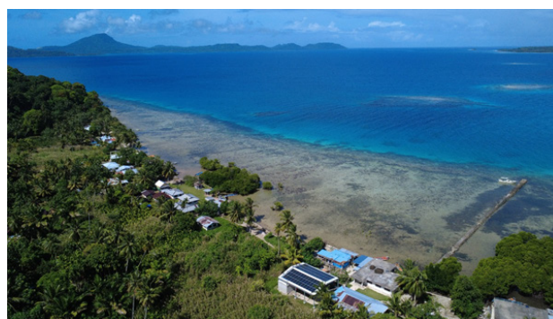
Figure 5. Solar mini-grid in Penia, Udot, Chuuk
