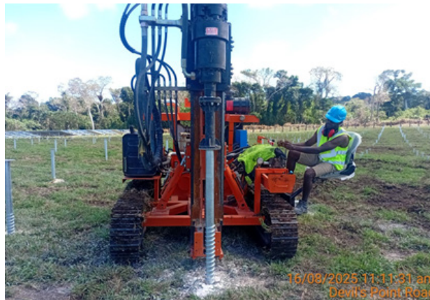
A total of 1,944 screw piles were installed using our own equipment to support fixed-tilt mounting structures under challenging ground conditions.
