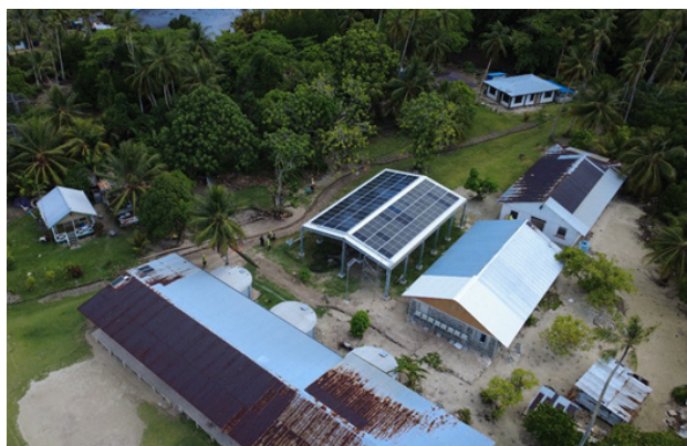
Figure 1. Mini-grid under construction in Eot, Chuuk
