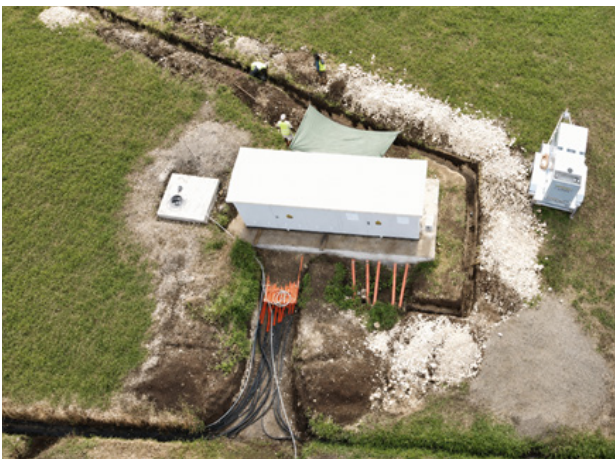
Civil and electrical works included trenching, cable installation, and integrated communications infrastructure.
