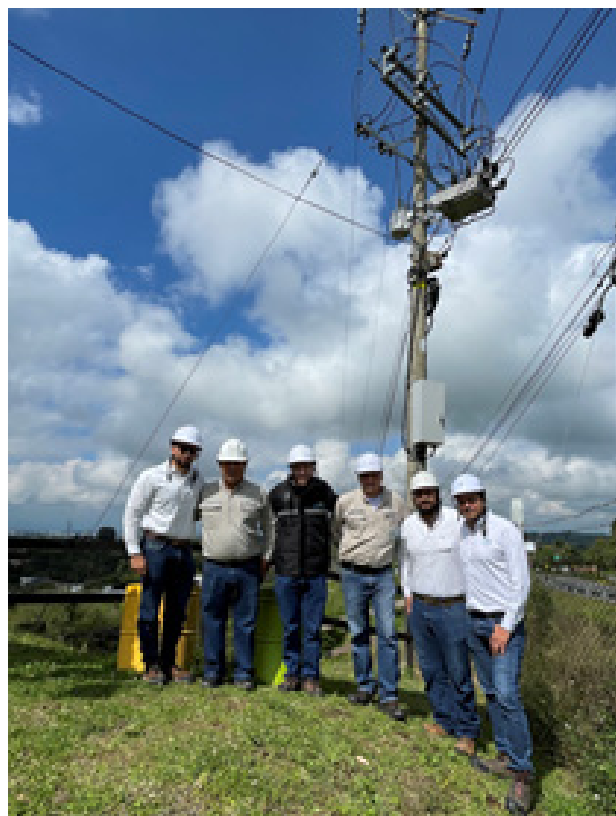
The EDEQ team with NOJA Power's OSM Recloser in a rural site in Quindío, Colombia.
