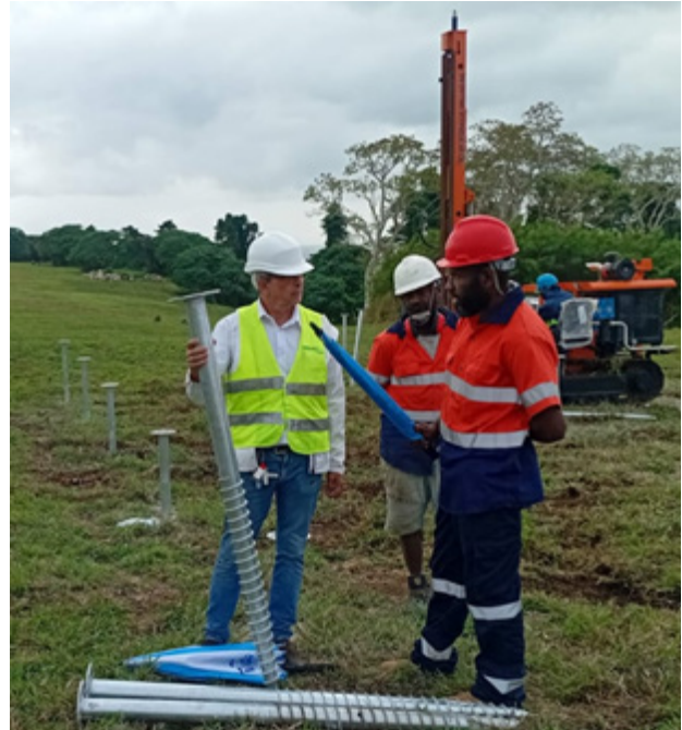
Close collaboration between PEP and UNELCO supported successful project delivery and commissioning - Tanguy Kerzreho of UNELCO Inspecting work in progress with PEP Site Manager Charles Mickey
