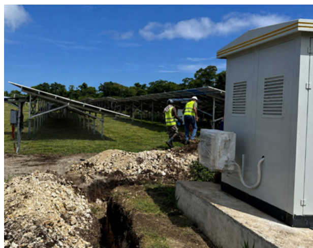
Rocky ground conditions required engineering adjustments to maintain installation integrity.
