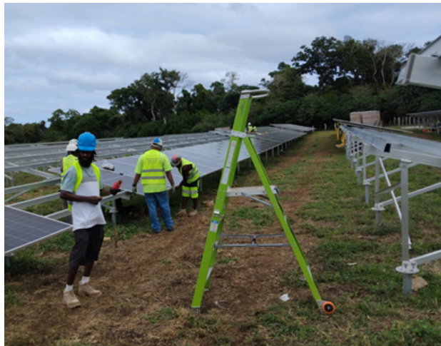
Installation of 4,320 high-efficiency PV panels formed a key stage of construction.
