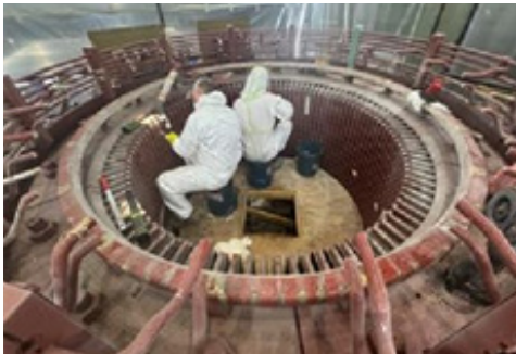
AW Team Preparing support rings & core for
