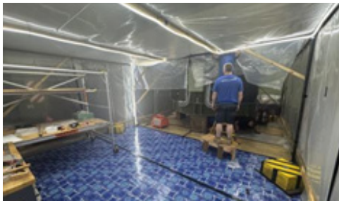
AW Makeshift Clean Conditions & FME Zone ready for rewind
