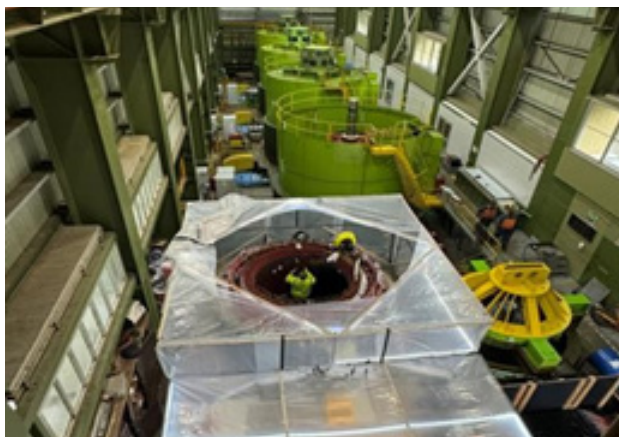
Bird's-eye view inside the makeshift controlled enclosure built on site to manage humidity, cleanliness and rewind conditions.
