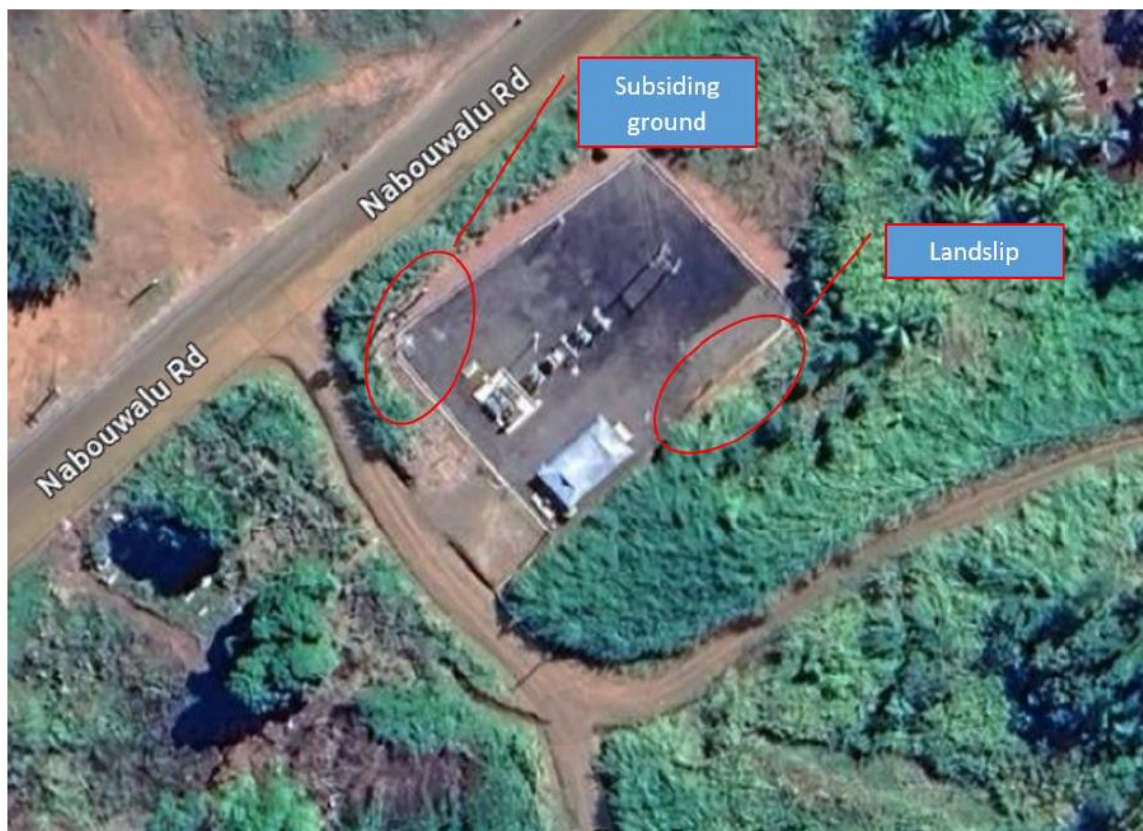
Fig.2 Dreketi 33kV/11kV Sub-Station and Area's affected by Landslide.
