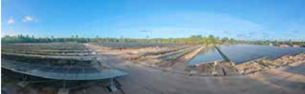
PhotoVoltaic Arrays nearing completion
