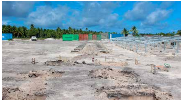
Early Days of Construction
