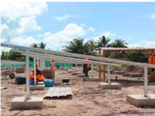
Early days of Construction
