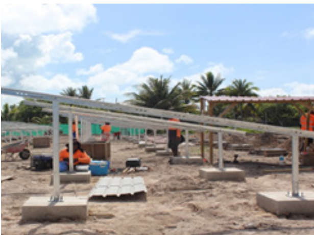
Early days of Construction
