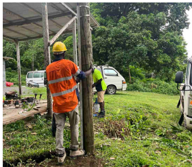
VanPAWA field crew in undertaking low-voltage network extensions to enable new customer connections and improve access to electricity in Malekula
