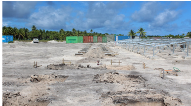
Early Days of Construction
