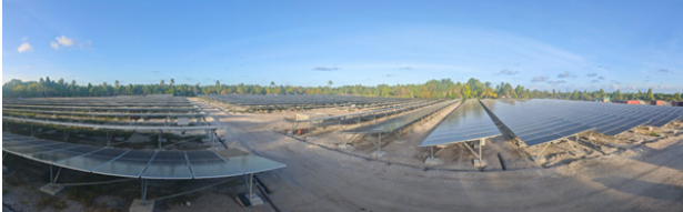
PhotoVoltaic Arrays nearing completion
