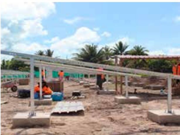
Early days of Construction
