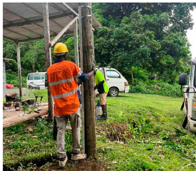
VanPAWA field crew in undertaking low-voltage network extensions to enable new customer connections and improve access to electricity in Malekula
