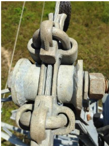
Figure 1.2: Existing OHEW assemblies – (Left: Suspension, Right: Strain)
