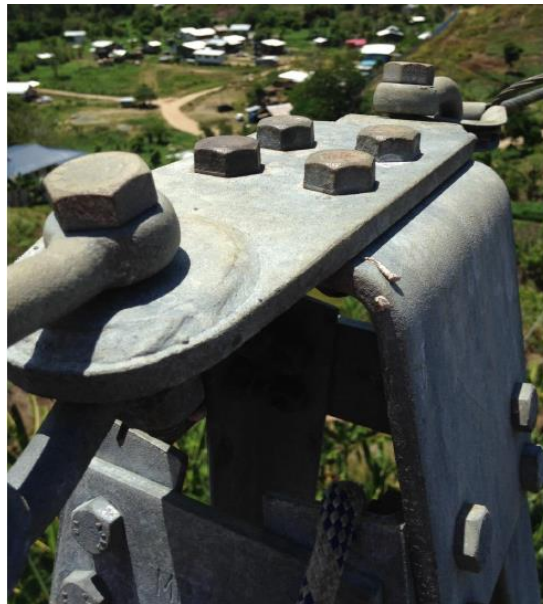
Figure 1.2: Existing OHEW assemblies – (Left: Suspension, Right: Strain)
