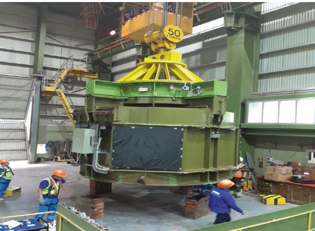
Stator positioning works
