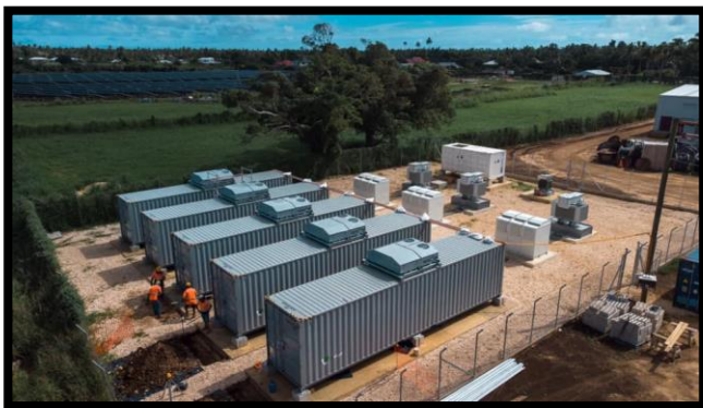
4-hour 'Storage' BESS (6 MW / 20 MWh) at a network feeder junction
