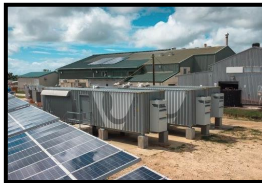
30-minute 'Power' BESS (7 MW / 4 MWh) at Popua Power Station
