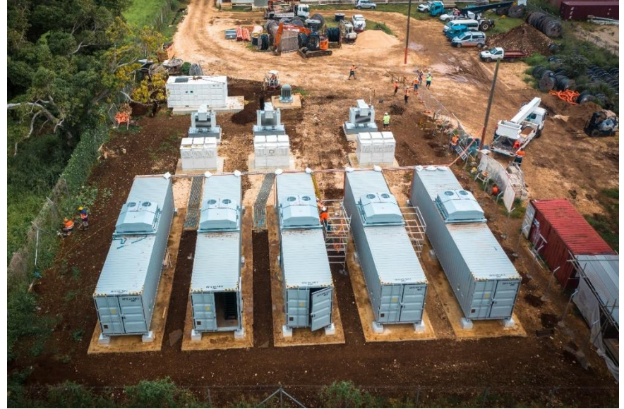
4-hour 'Storage' BESS (6 MW / 20 MWh) at a network feeder junction and co-located solar farm
