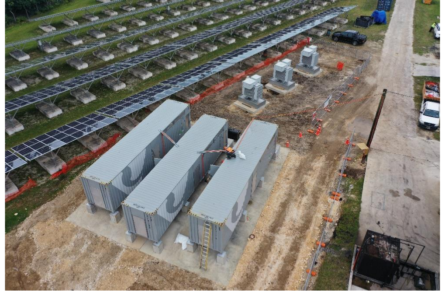
30-minute ‘Power’ BESS (7 MW / 4 MWh) at Popua Power Station
