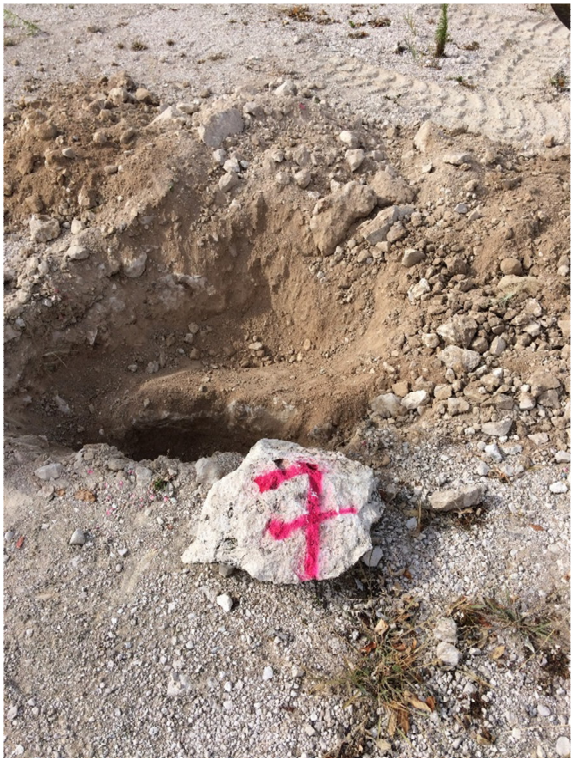
Test Pit 7 (Total Depth = 500mm)
