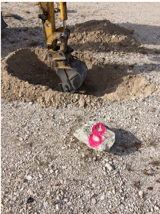
Test Pit 8 (Total Depth = 1600mm)
