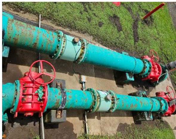
Figure 6-7: Tafuna WWTP - Effluent Magmeters
