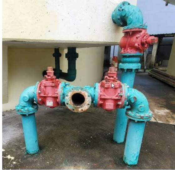
Figure 6-34: Utulei WWTP – Sludge draw points from the Clarigester 2 and 3
