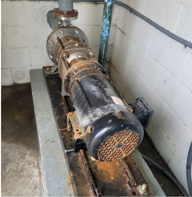
Figure 6-13: Tafuna WWTP – Booster Pump for Utility Water System
