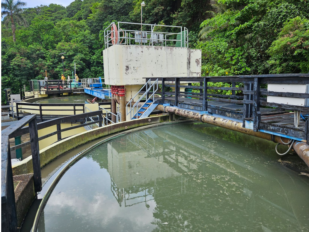
Figure 6-30: Utulei WWTP – Elevated Splitter Box and Clarigesters
