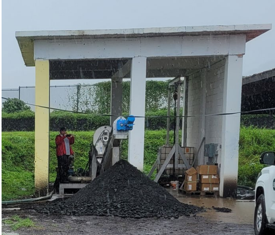
Figure 6-11: Tafuna WWTP – Screw Press
