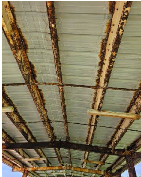
Figure 6-9: Tafuna WWTP – Corrosion of the Metal Covering the UV Channels
