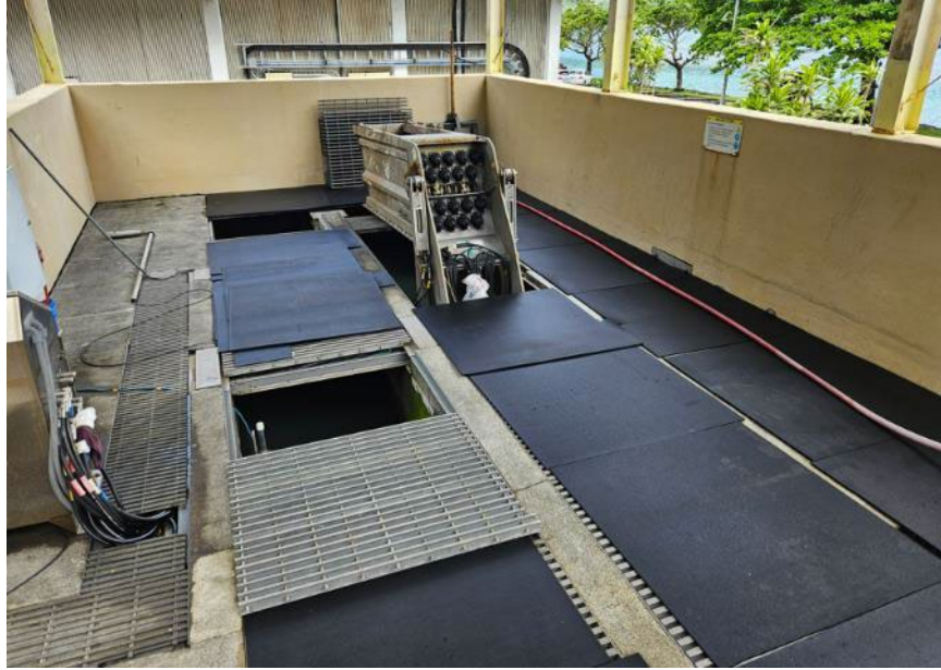
Figure 6-32: Utulei WWTP - UV Disinfection Unit
