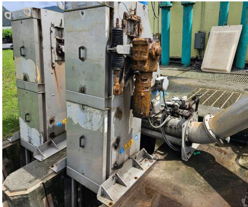
Figure 6-5: Tafuna WWTP – Screens in Parallel Channels
