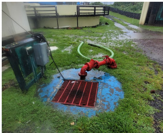
Figure 6-14: Tafuna WWTP – Plant Drain Lift Station
