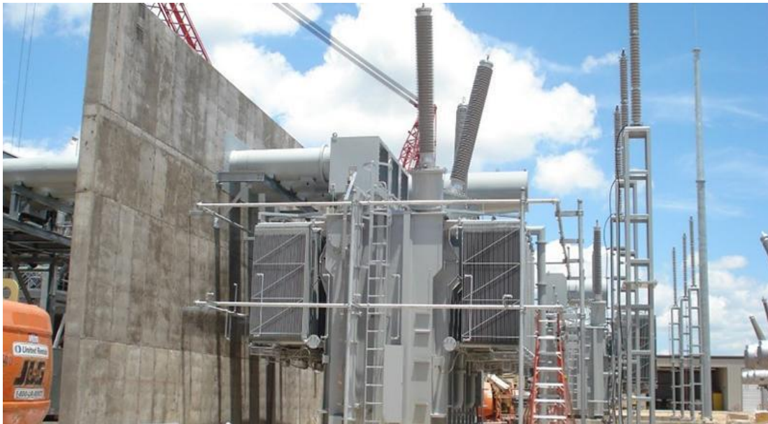
Figure 7-4 Transformer Fire Protection System with Fire Wall
