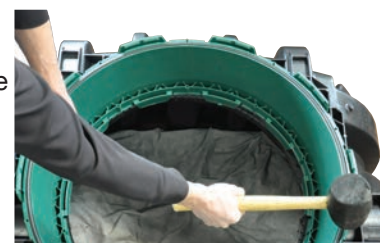
Use mallet to engage the rest of the tabs.
