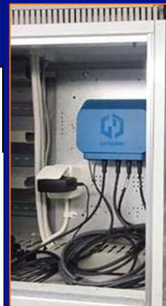
Fig. 17 – 'Grayfox' for the UG cable network has Rogowski sensors attached to cable screens.
