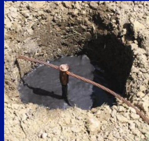
Fig. 12 - Patented Eritech 'Hammerlock' connector
