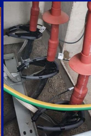
Fig. 18 – The integrated 'Safegrid' solution offers the precise location of faults, full network visibility, enables predictive maintenance, and improves SAIDI/SAIFI. Ideal distances between sensors in a rural area are 4 to 10km with a fault location accuracy of <200m.
