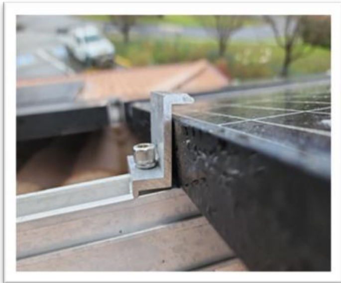
(1) wrong size end clamp used (2) PV cables pinched
