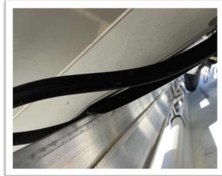
(1) wrong size end clamp used (2) PV cables pinched
