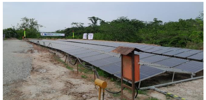
Figure 4: "Solar Wings" Deployment from a solar containers Mobil-Grid® 72 kWp
