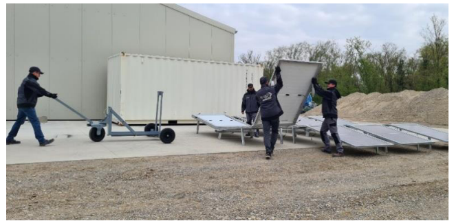
Figure 4: "Solar Wings" Deployment from a solar containers Mobil-Grid® 72 kWp
