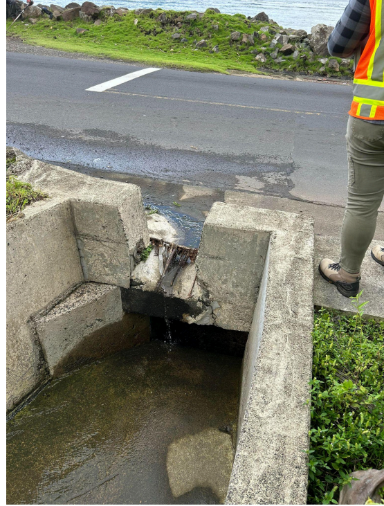
Stormwater box culvert #1 before Tutuila Store - Leloaloe
