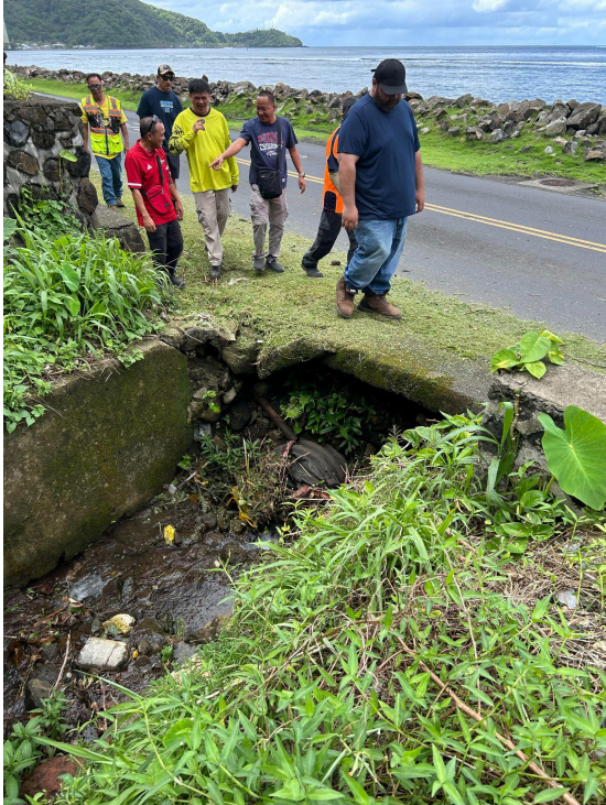
Plastic SD culvert pipe next to Leloaloe Catholic School
