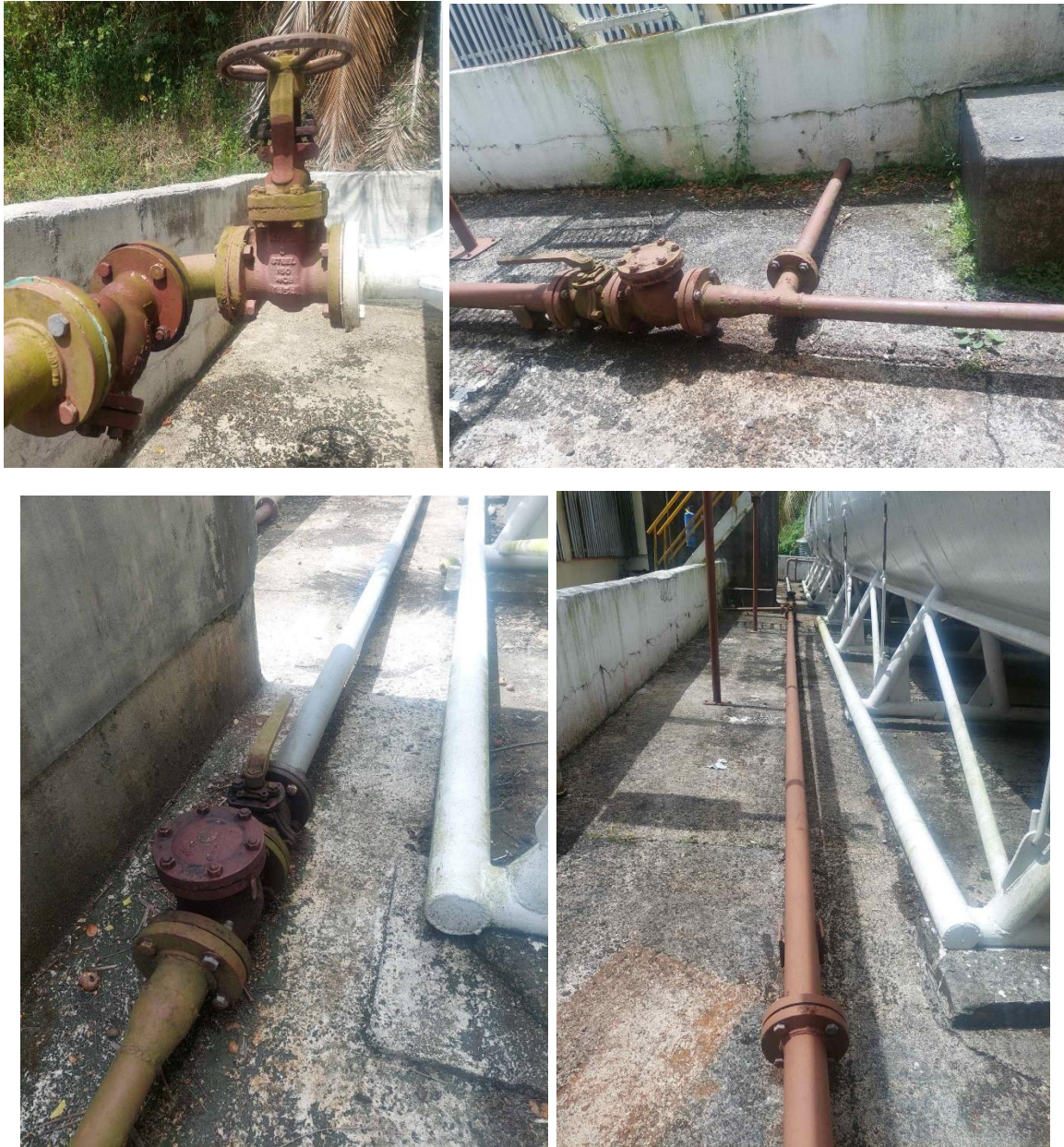
Figure 1: 3" discharge line in tank bund
