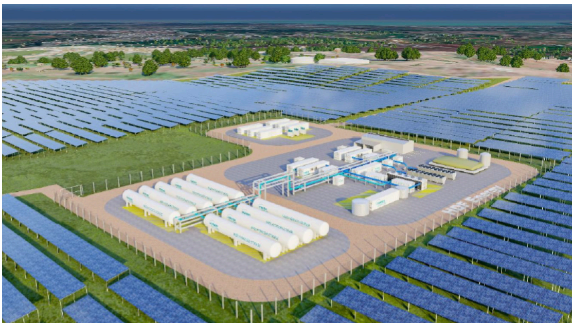
Figure 2: Overview of the process area of the Viti Levu Renewstable® Power Plant..
