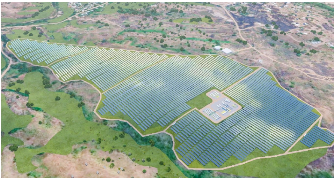
Figure 1: Illustration of the Viti Levu Renewstable® power plant.
