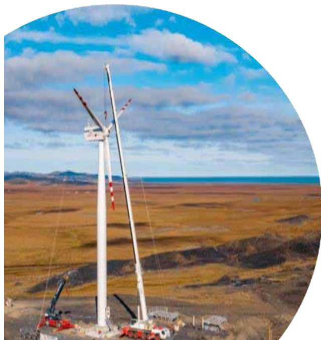
Picture 1. KWT300 Rotor Hub Installation
