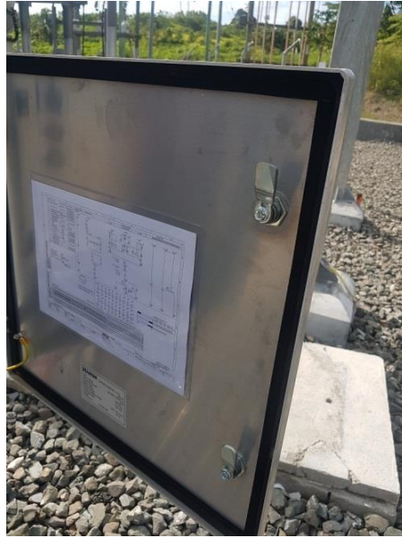
Figure 6: Rubber Installed on doors to prevent water and insects entering
