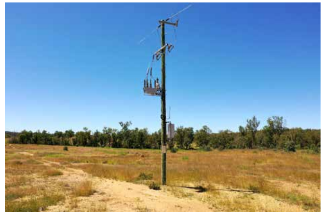
A Single Wire Earth Return network with a NOJA Power OSM Recloser
