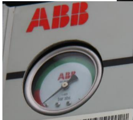
Photo 30: 11 kV RMU with SF 6 Gauge on Zero
