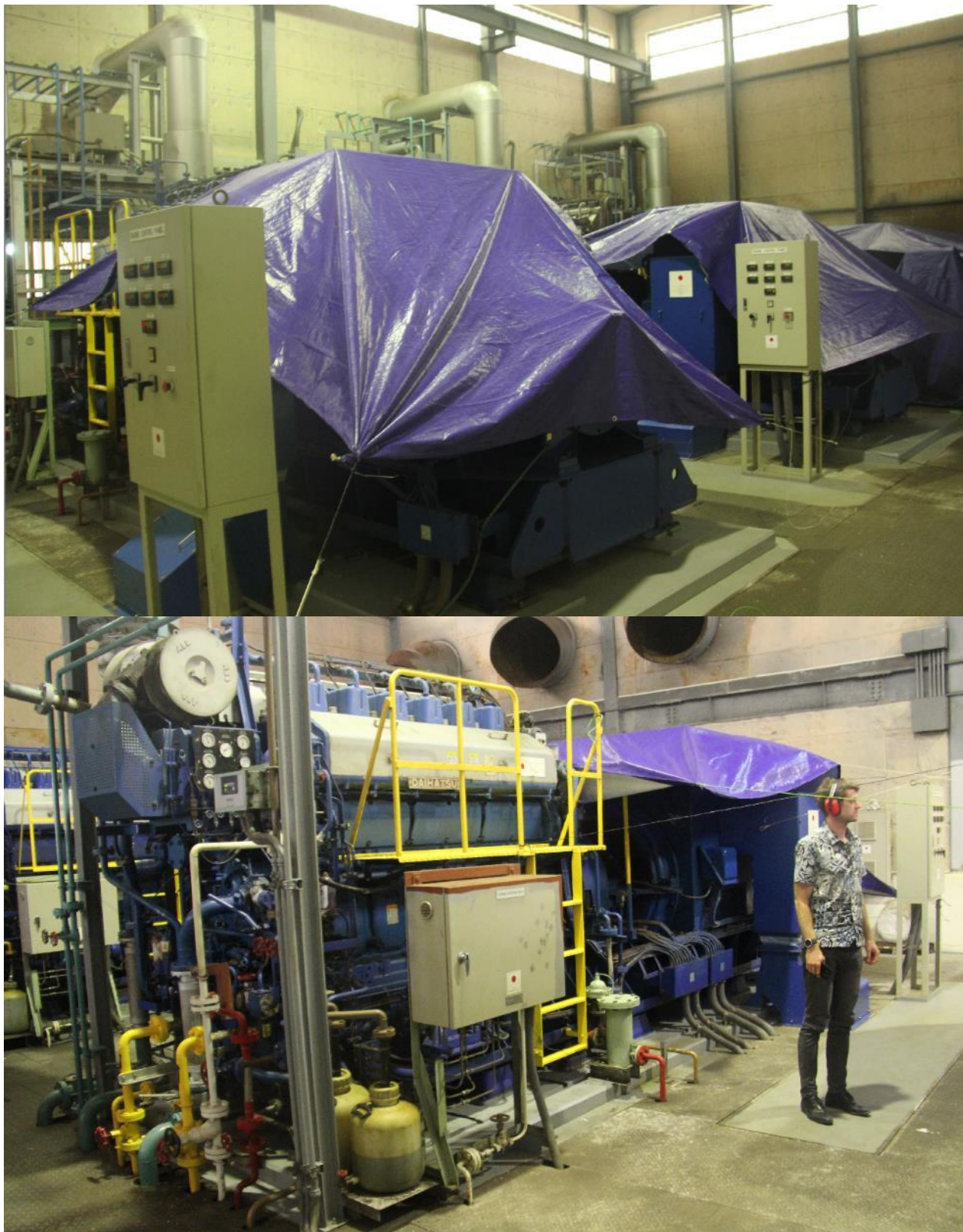
Photo 20: Funafuti Power Station - Alternators Protected from Rain
