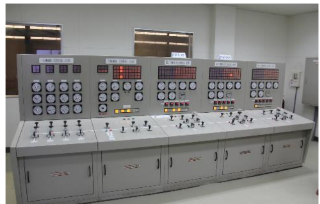
Photo 23: Funafuti Power Station - Control Panel and Control Desk
