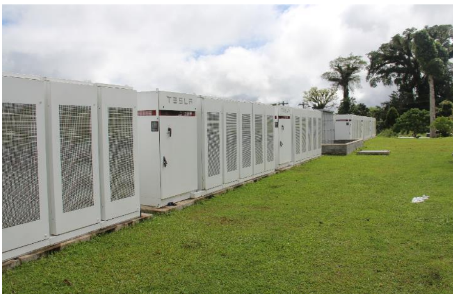
Photo 5: Fiaga Power Station BESS
