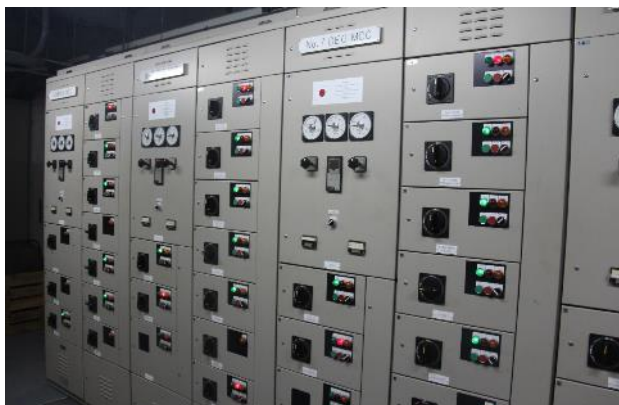
Photo 23: Funafuti Power Station - Control Panel and Control Desk
