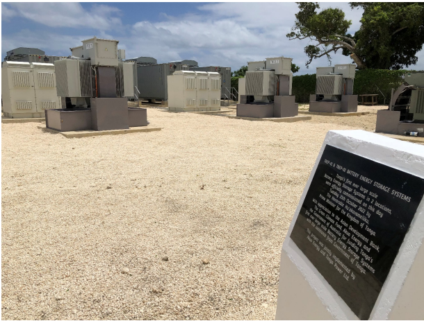
Load-Shifting battery: 23MWh/7MW
