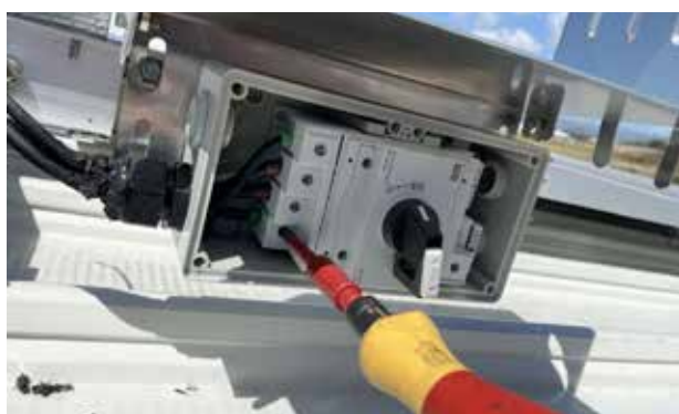
Figure 10 - Torque being checked at a terminal. Always make sure you have tightened all your connections to the manufacturer's specification.
