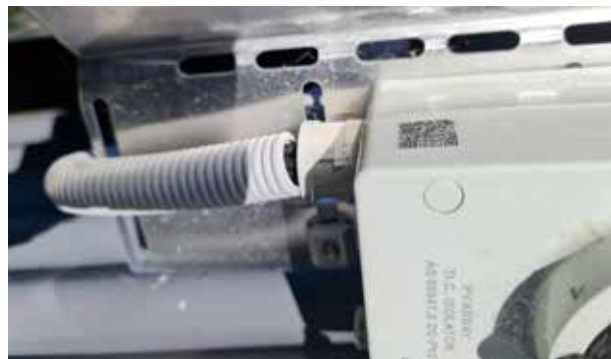
Figure 4 – Conduit not glued and falling out of the adaptor. Conduit must be glued to ensure watertightness and steadfastness at the connection.
