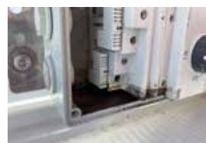
Figure 3 – partial immersion of the isolator and corrosion evident with watermark and presence of green - copper conductor corroded, and brown - iron screw corroded
