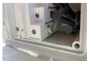
Figure 2 - evidence of corrosion at an isolator terminal
