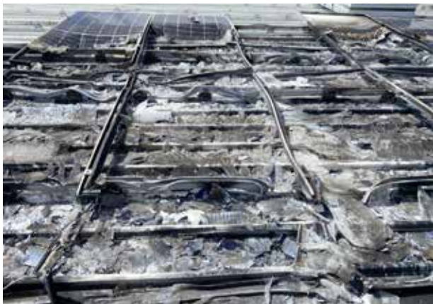
Figure 1 - Fire damaged array. Solar fires are headaches for the owner and the installer
