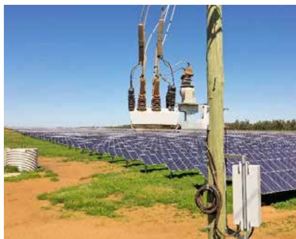
A NOJA Power OSM Recloser connecting Renewable Generation Energy to the Distribution Grid
