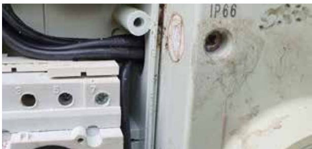
Figure 7 - penetration of an enclosure without appropriate sealing and not utilising the lower surface.
