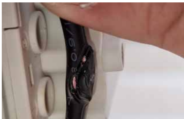
Figure 11 - DC cable pinched by enclosure lid.
