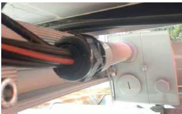
Figure 6 - single hole compression gland used for multiple cables entering the gland.
