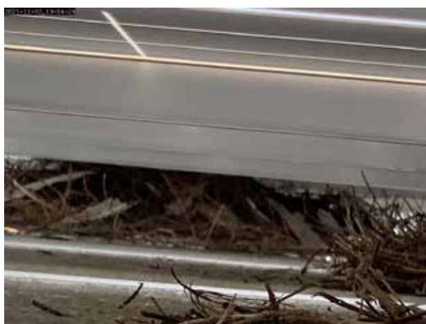
Figure 15 - Vegetation build-up under panels due to bird nesting. Gutter guards can be installed around the modules to prevent debris build-up and fauna access.
