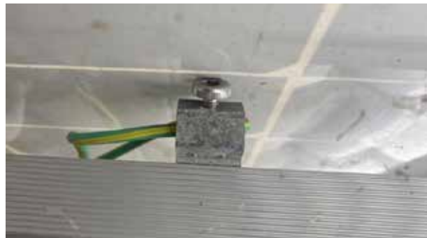
Figure 12 - earth lug installed hard against the underside of the module]
