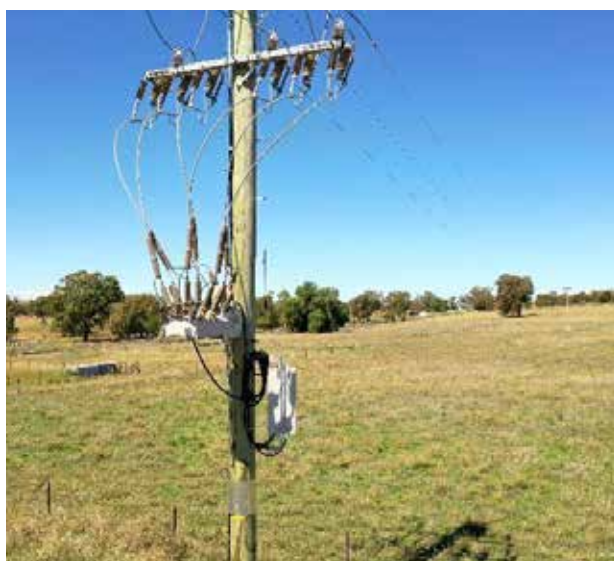
A NOJA Power OSM Recloser protecting Overhead Lines
