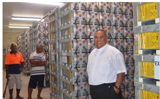
Battery Storage at Outer Islands of Nanumea.
