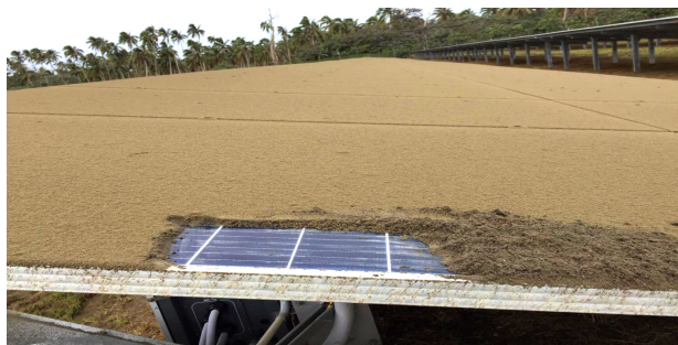
Heavy ash deposits covering solar arrays
