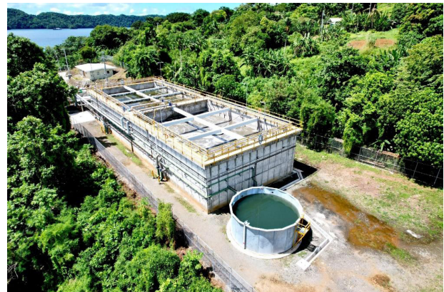
Malakal Sewer Treatment
