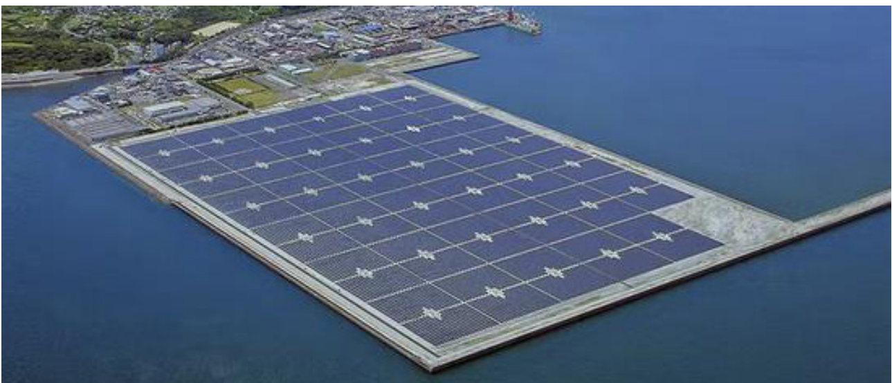
Kagoshima PV, Japan (Source: John Major, Univ of Liverpool)
