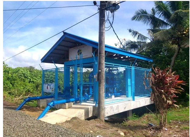
Ngerikiil Pump Station
