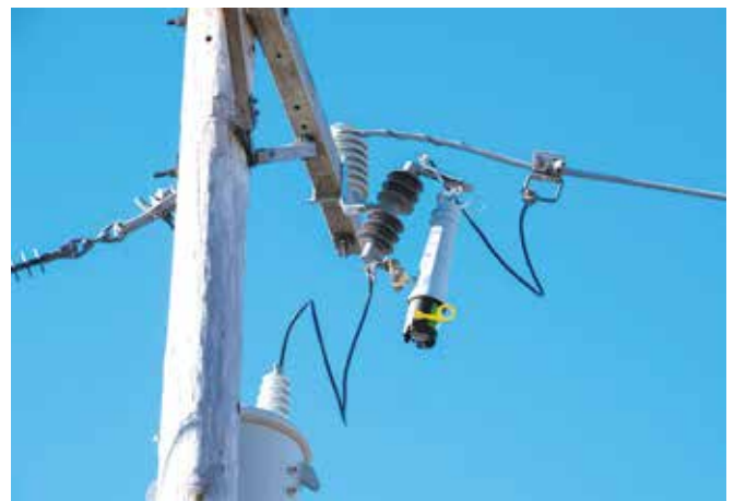
S&C's VacuFuse® II Self-Resetting Interrupter.
