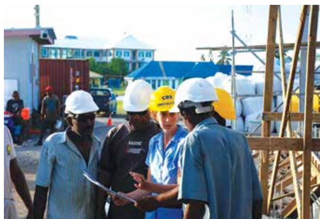
CBS Site Manager during construction of the TEC solar plant in 2015
