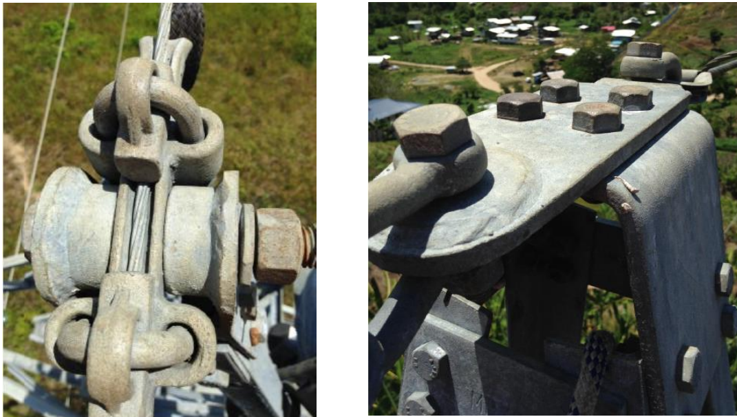
Figure 1.2: Existing OHEW assemblies – (Left: Suspension, Right: Strain)
