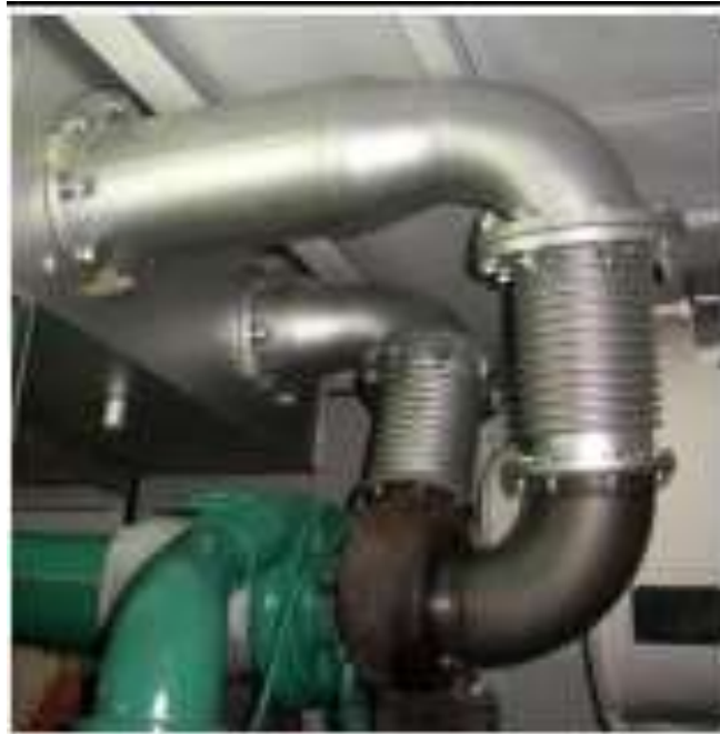
Figure 1 Exhaust Bellow
