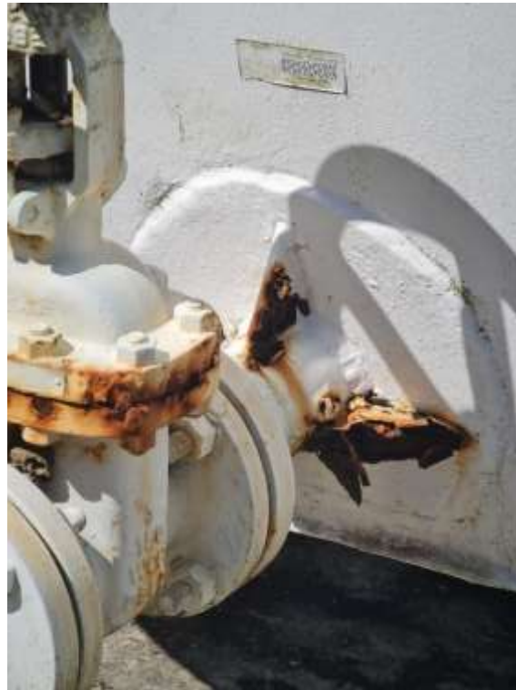
Figure 4 Discharge nozzle on Tank 2
