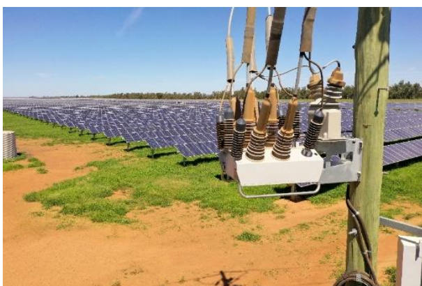
A NOJA Power OSM Recloser used as the point of connection switchgear for a Grid Scale Solar Farm
