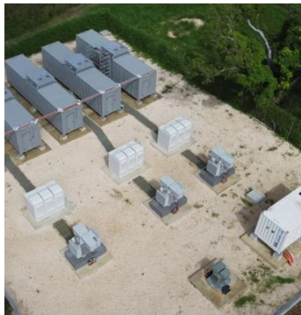
Figure 2 Load Shifting BESS installed behind TPL's headquarters on Tongatapu
