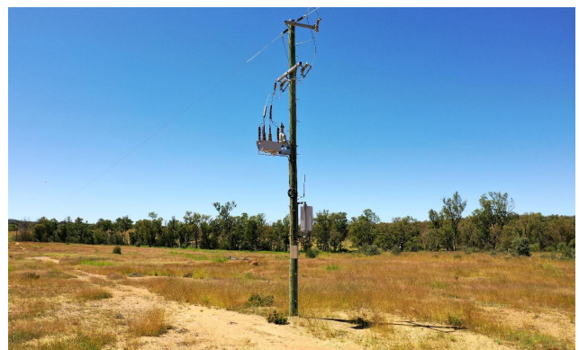
A Single Wire Earth Return network with a NOJA Power OSM Recloser
