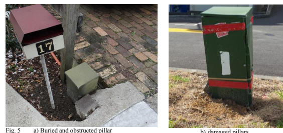
Fig. 5 a) Buried and obstructed pillar
