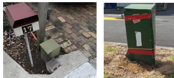
b) damaged pillars
