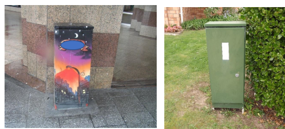
b) Link pillar in the urban green space near a park with the bottom open and accessible to the public, creating a safety hazard, especially for children playing around.
