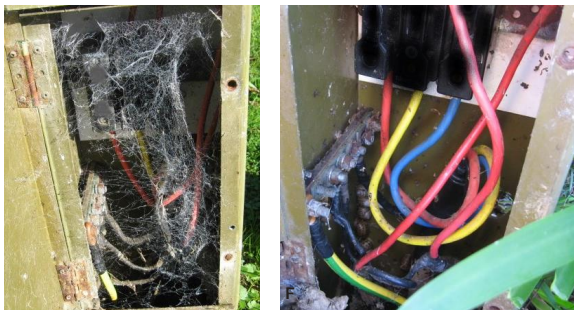
Fig. 3. Rusty hinges and internal parts of metal service pillars, caused by moisture and daily thermal cycle
