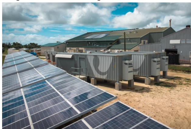
Figure 1 Grid Stabilizing BESS at the main Diesel Power Plant on Tongatapu
