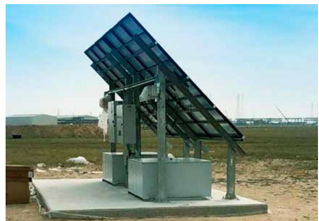
Solar electric array with Morningstar controllers powering oilfield lighting in the desert, for Kuwait Petroleum Corporation. Courtesy EcoSol Energy Systems
