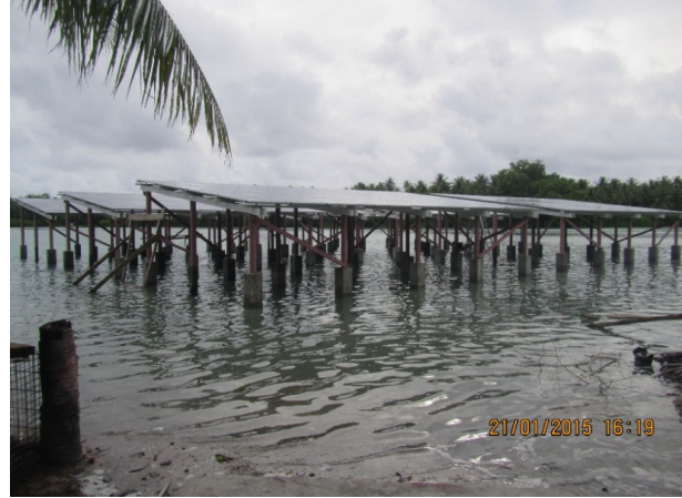
PV Modules – Structure in the Estuary
