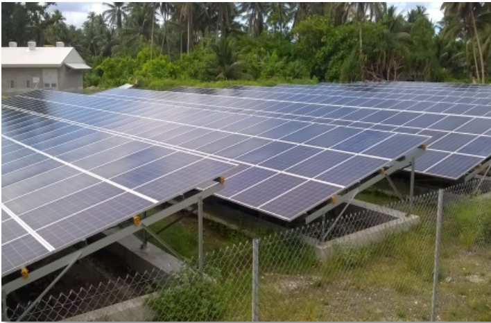
PV Modules – Ground Mounted
