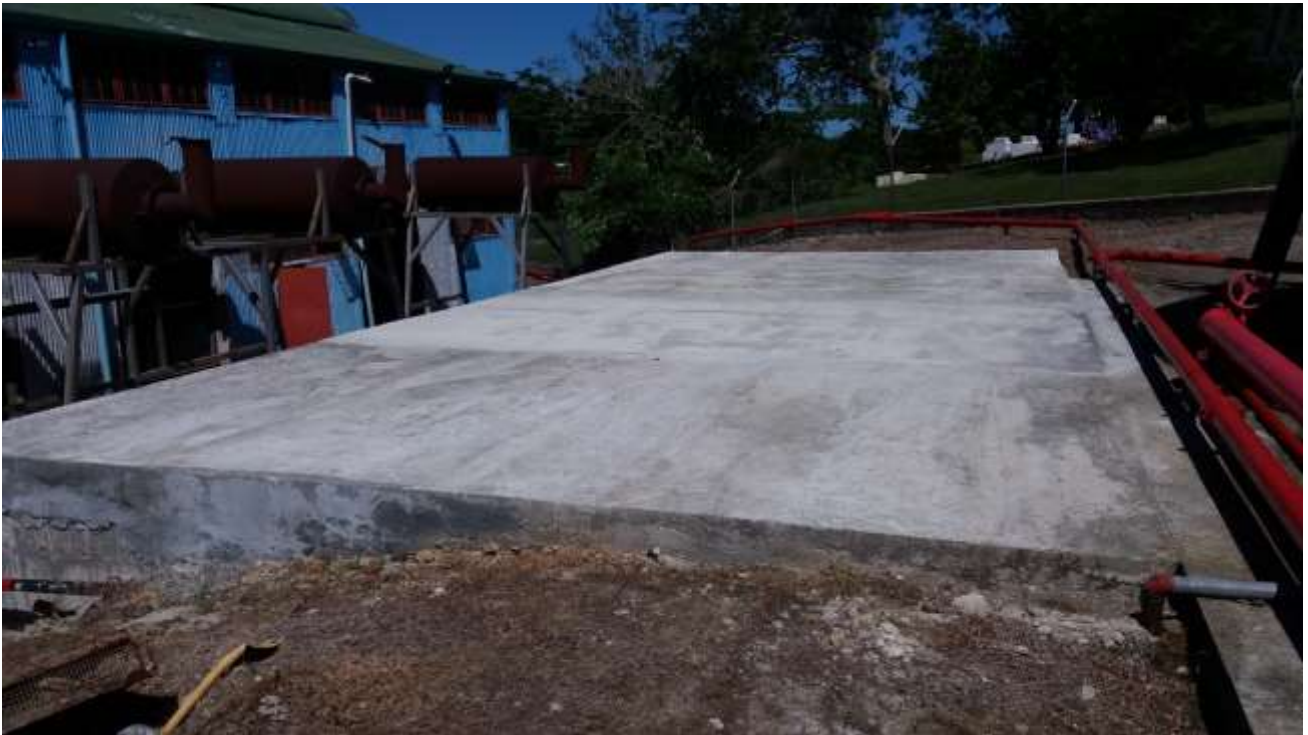
Figure 1: View of Concrete Pad for Remote Radiator Installation.
