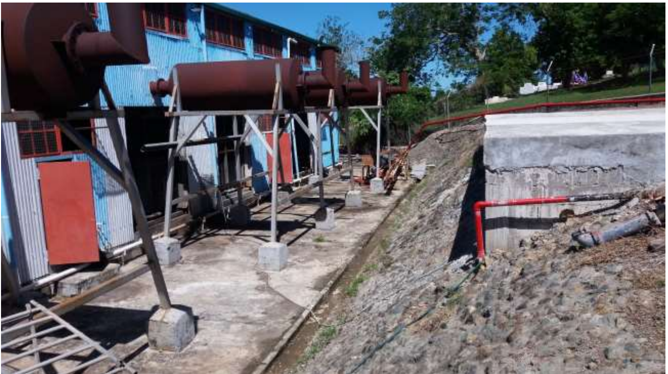
Figure 2: View showing height difference between Concrete Pad and Generator Floor (approx.3m).
