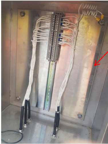
FIGURE 3.1 – Pan Installed/bolted in Box
