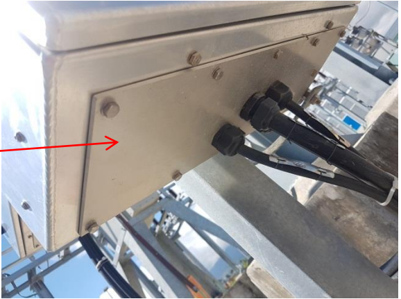
FIGURE 3.2 – Gland Plates Installed in Box
