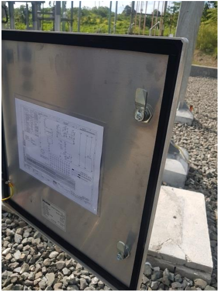
FIGURE 3.3 – Rubber Installed on doors to prevent water and insects entering
