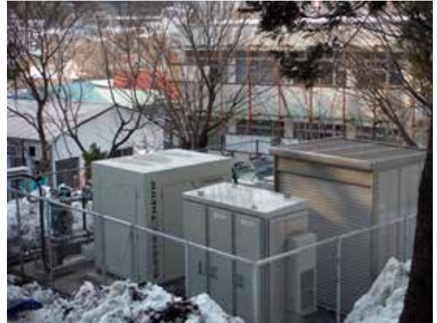
ORC Installation Central Japan
