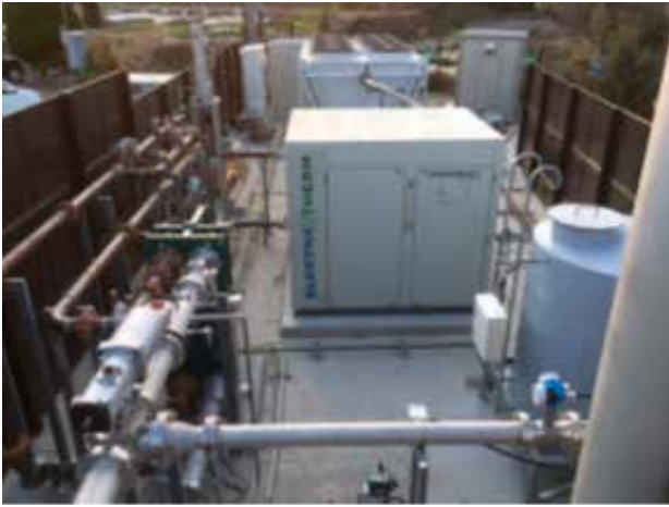
ORC Installation at Beppu Japan
