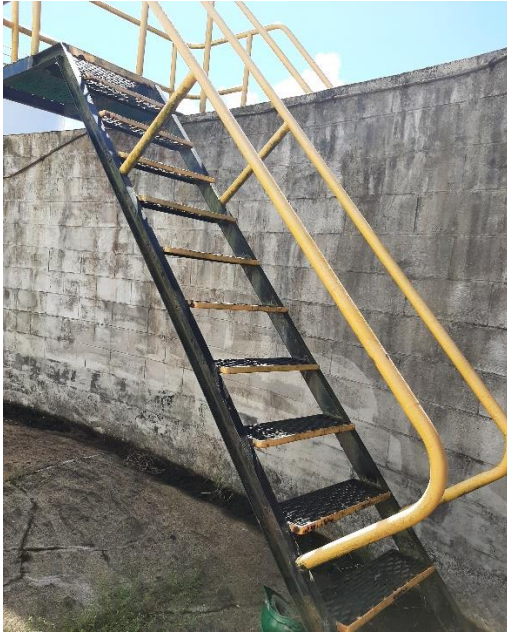
Figure 1: Bund wall Stairway
