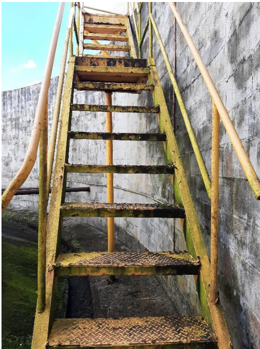
Figure 5: Bund wall stairway
