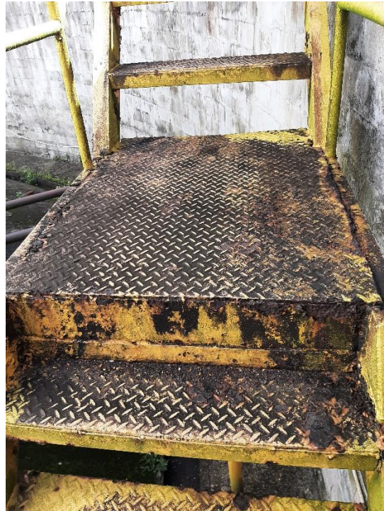
Figure 4: Bund wall stairway
