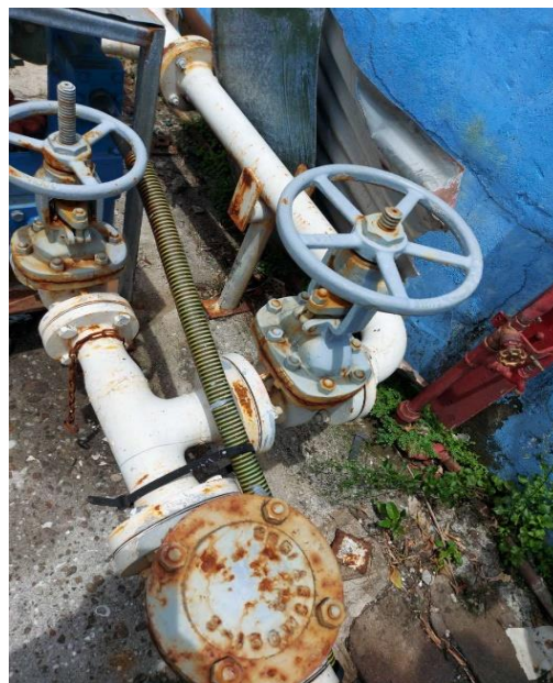
Figure 4: Fuel supply valves
