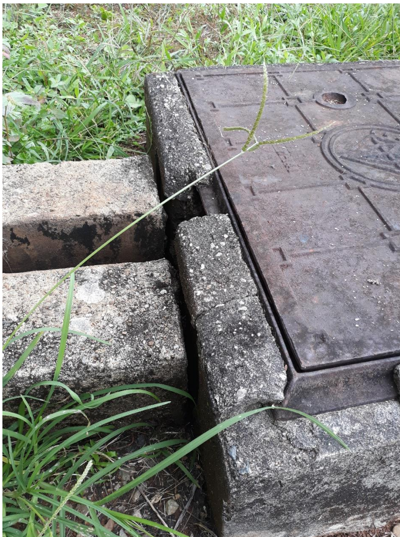
Figure 1 Inlet of Oil Interceptor
