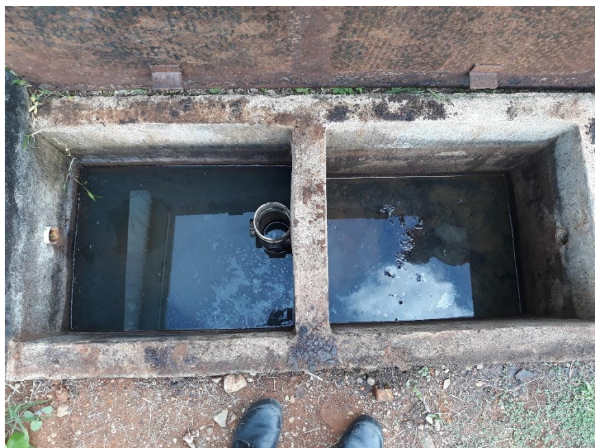
Figure 3: Interior 2 stage interceptor
