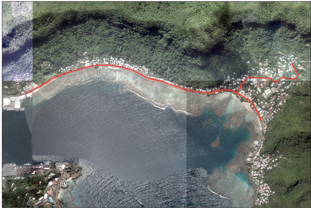
AUA AREA ACP REPLACEMENT
