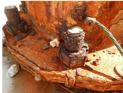
Figure 2 Decay of the basement of the old antenna tower
