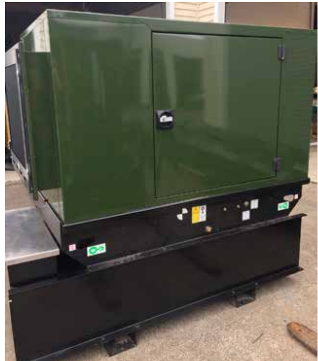
Base Tank with Generator
