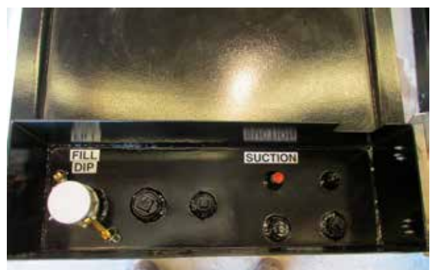
Aerial view of fill ports for Terra Cat base tank
