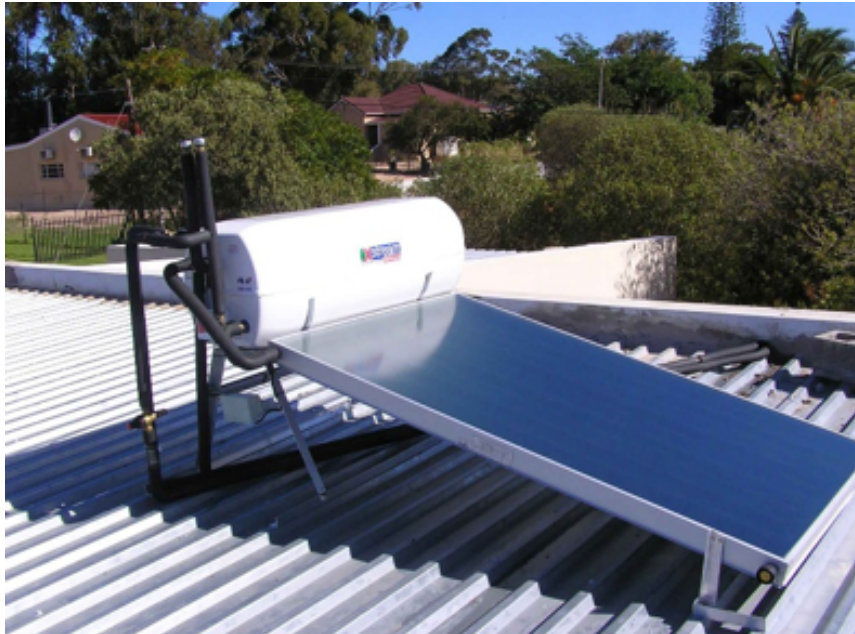
Figure 13: Typical Installation On A Flat Roof
