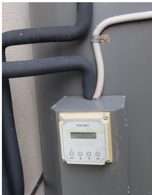
Figure 28: Controller & Pump Securely Attached To The Tank Jacket
