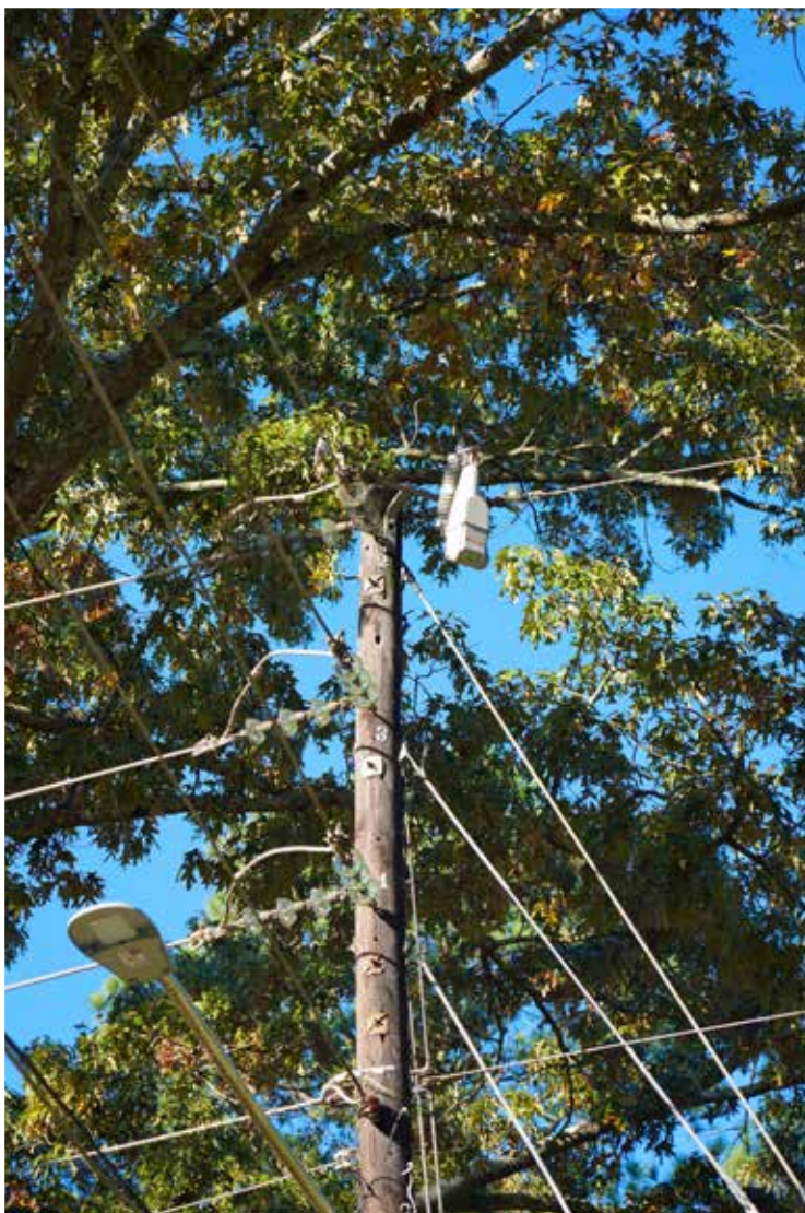
Top - S&C's TripSaver® II Cutout-Mounted Recloser in three-phase, group operations configuration
