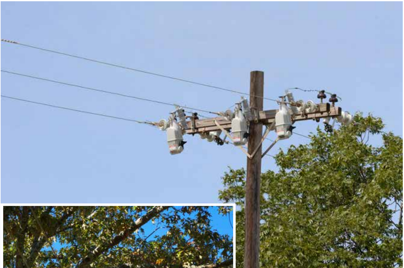
Top - S&C's TripSaver® II Cutout-Mounted Recloser in three-phase, group operations configuration
