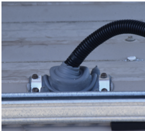
Figure 16: A Dektite® with a metal roof flashing
